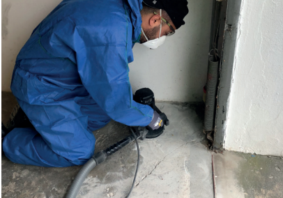
1. Subsurface preparation Grinding and vacuuming of the substrate.
