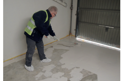
3. Applying primer Apply ASODUR-SG2 by brushing and rolling.
