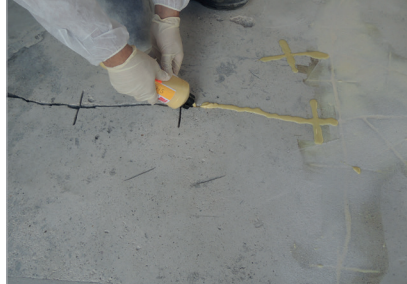
2. Crack repair With ASODUR-GH-S and subsequent sanding.
