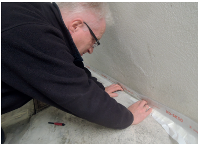
4. Applying the edging strip Apply RD-SK50 to prevent sound and mortar bridges.
