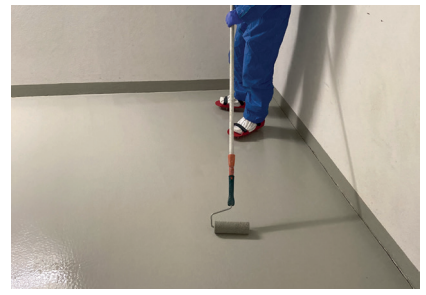
6. Top seal Apply ASODUR-V360W crosswise with a roller.
