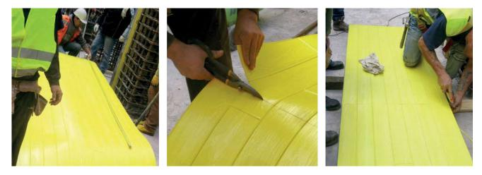
3. Different techniques can be used to fix the Strukturmatten.
