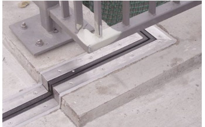
Refurbishment pedestrian bridge, Eilenburg, Germany
