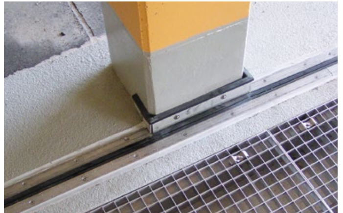
Parking garage Annaberg, Germany – FP 90
