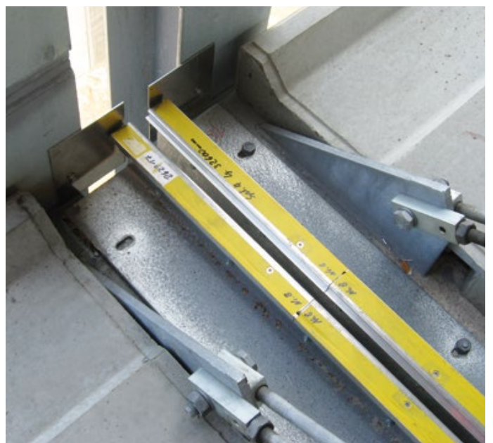
Parking garage Weiterstadt, Germany – FP 90
