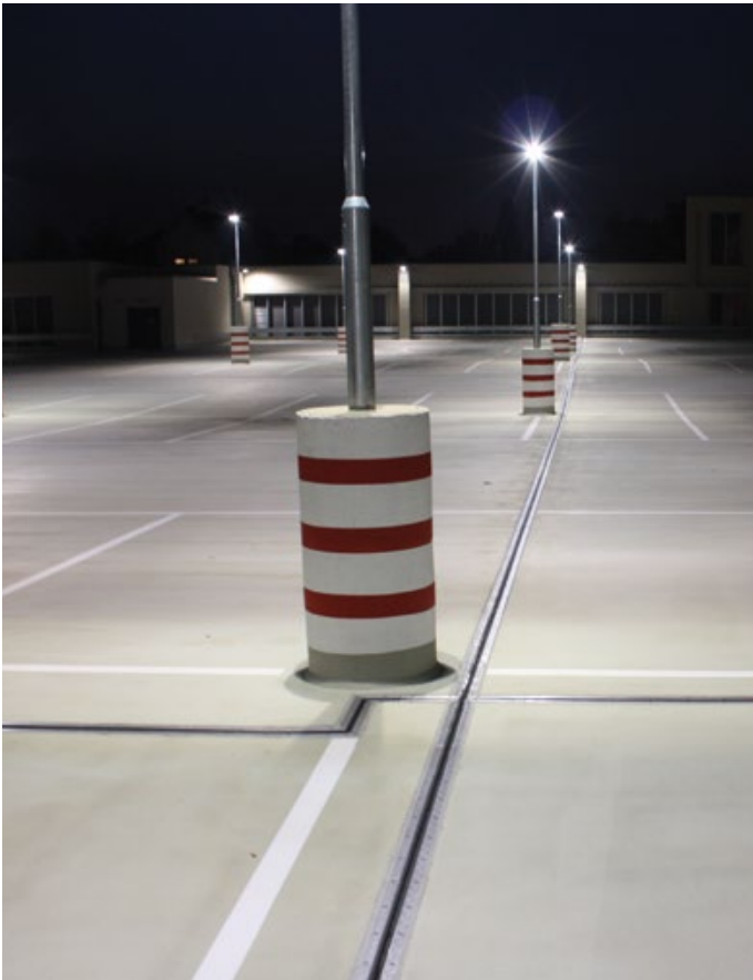
Parking deck shopping mall Dresden, Germany
