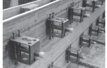
HSD-CRET sliding sockets nailed onto the formwork
