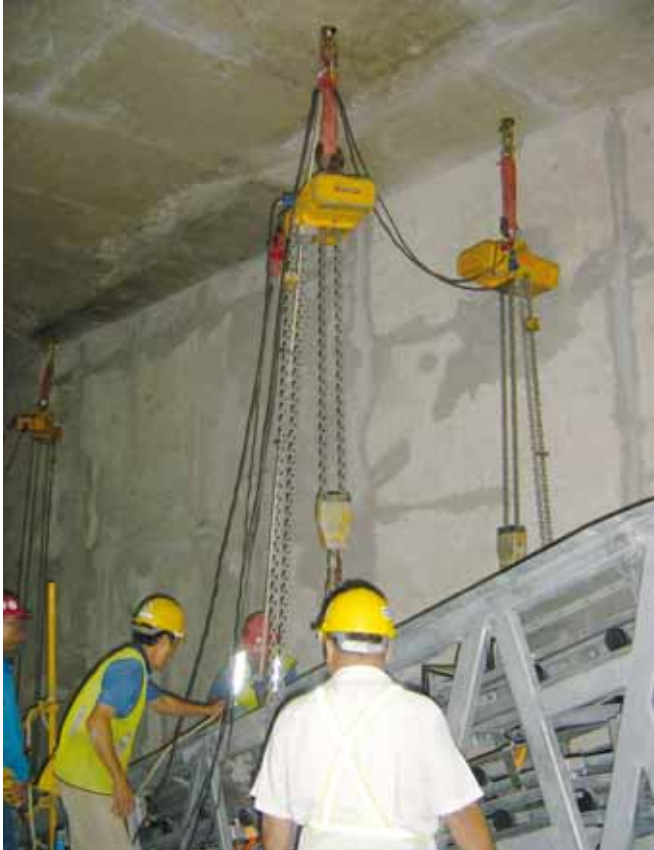
Typical setup for an overhead anchor system Multiple anchors used together to lift heavy equipment
